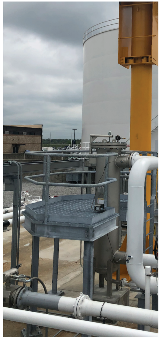
Figure 1. Magnetic separator installed upstream of tankage at airport fuel facility.
