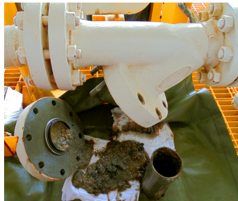
Figure 11: Y-strainer plugged off with black powder.
