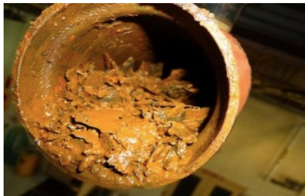
Iron oxide rust contamination built up in piping resulting from black powder.
