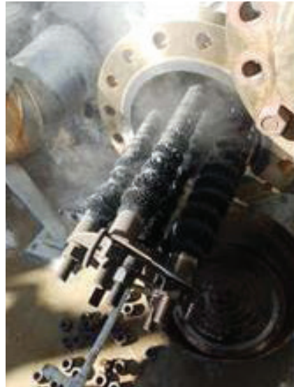
Figure 2. Removal of Magnetic Separator elements.
